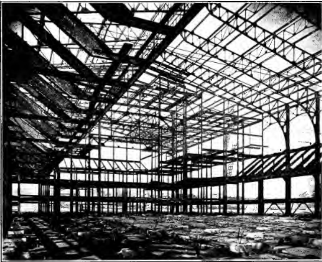
SHOWING HEAVY STRUCTURAL STEEL CONSTRUCTION OF OAKLAND AUDITORIUM
